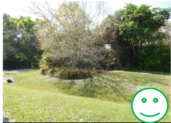
Clean swale and driveway culvert
